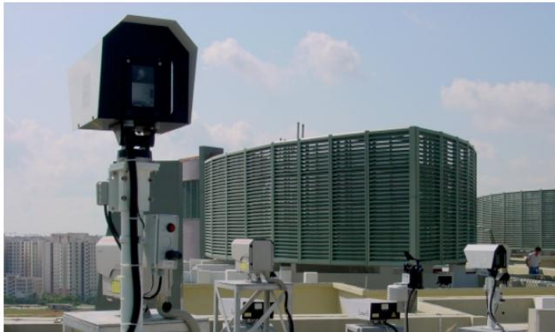
Fig: 6. Setup of FSO units in iDA test bed in Singapore
