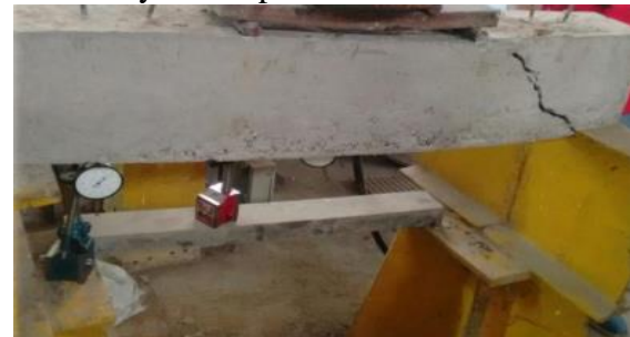
Fig.10. Beam BR1 at ultimate load
