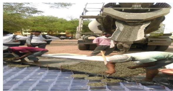
Fig. 8 Laying of Concrete.(Dagwal et al)
