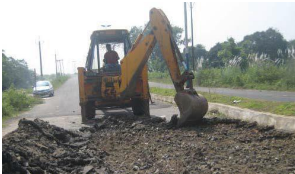
Fig. 4 Excavation of existing pavement.(Y.A.Singh et.al)
