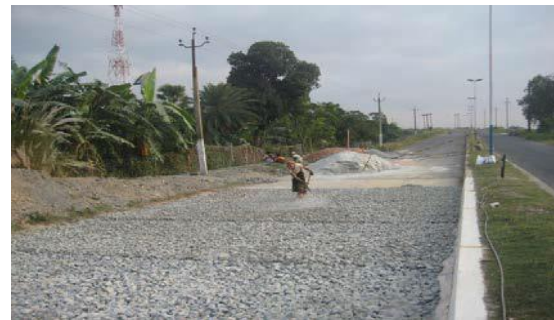
Fig.5 Laying and Compaction of sub-grade. .(Y.A.Singh et.al)
