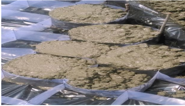
Fig.9 Compaction of Concrete. .(Dagwal et al)
