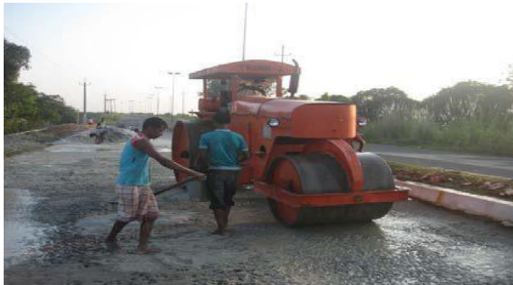
Fig.6 Laying and Compaction of sub-grade.(Y.A.Singh et.al)
